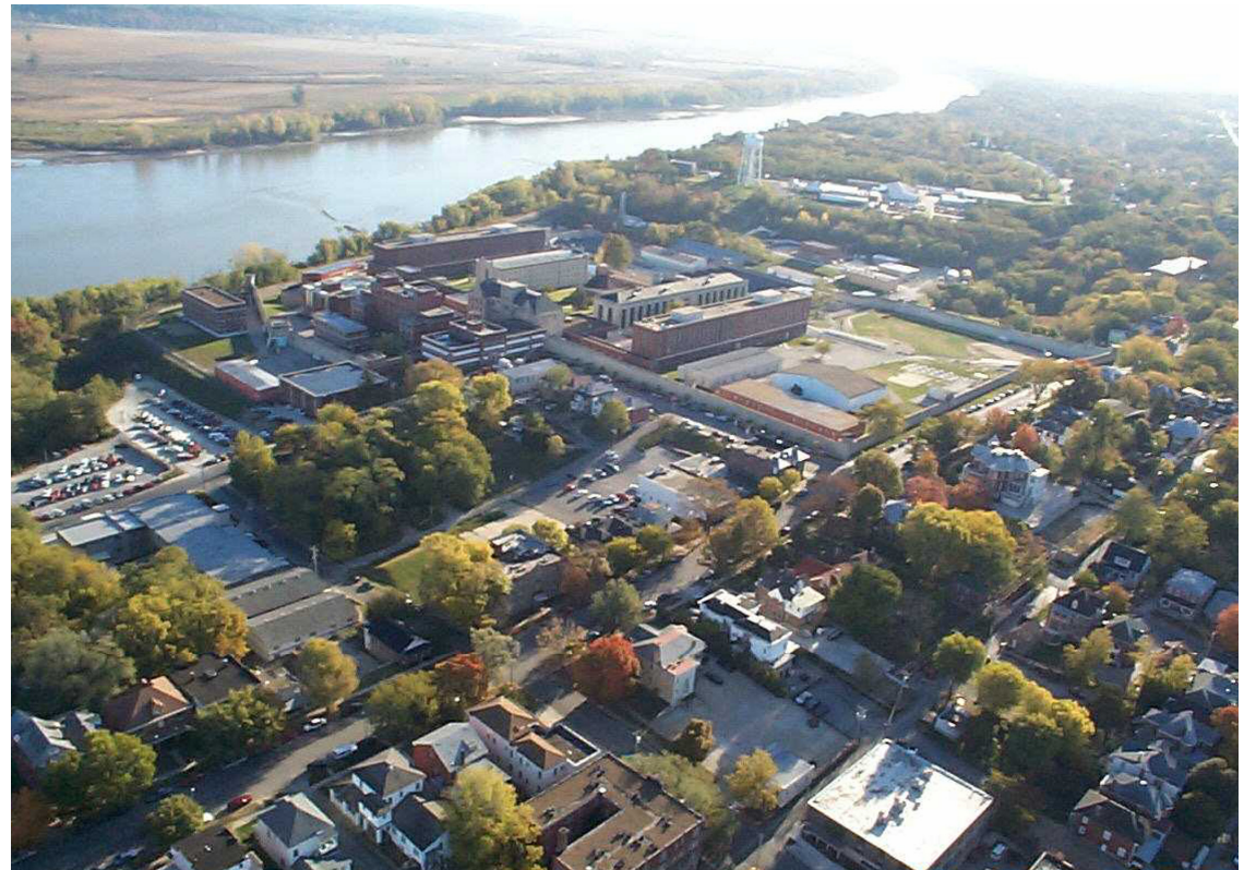
View of JCCC Looking to the Northeast
